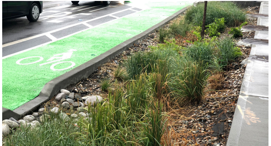
Before Rain Storm
