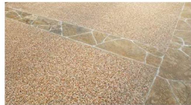
Exposed Aggregate Paving
