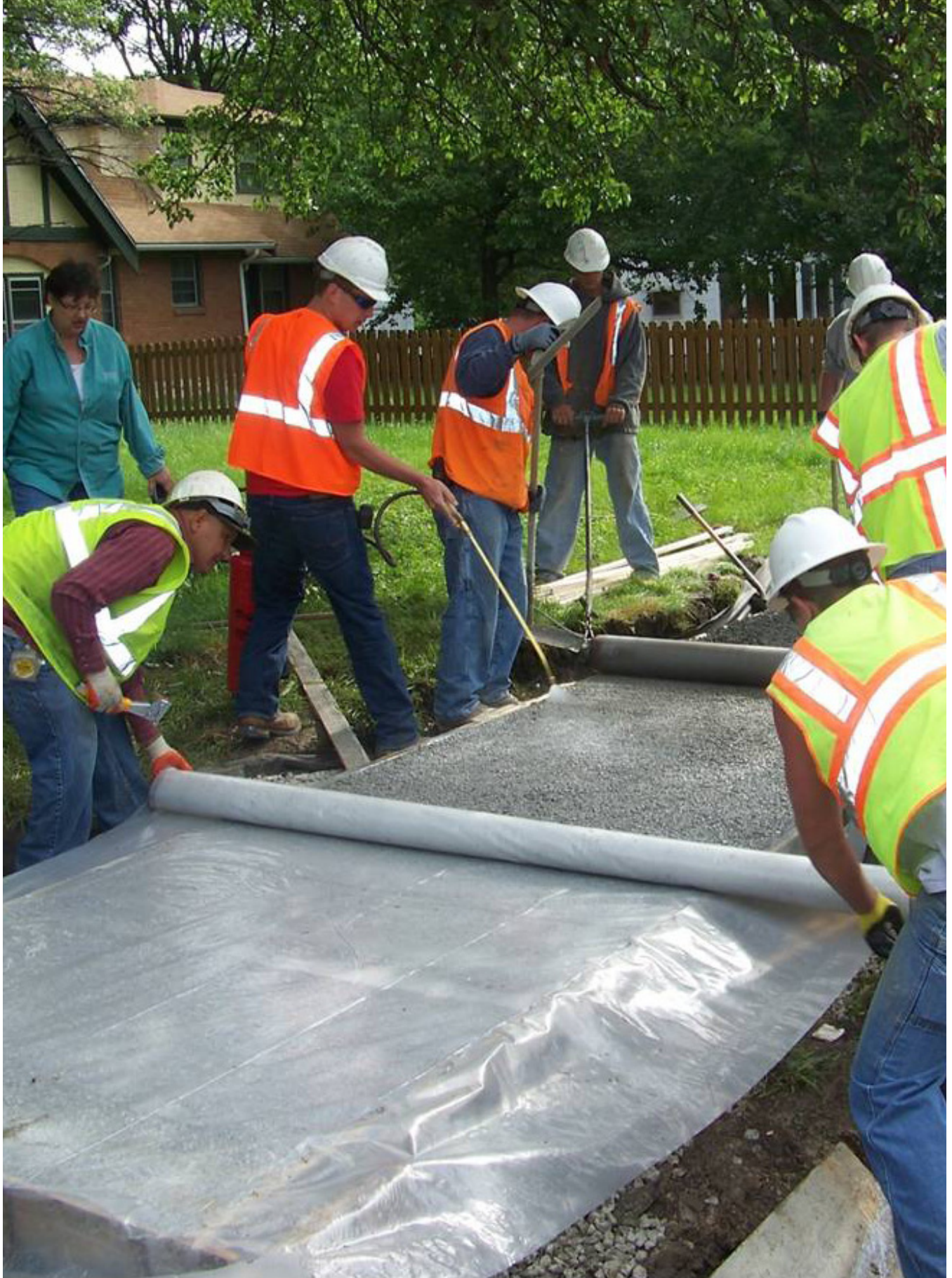
Porous concrete sidewalk, Middle Blue River Basin Green Infrastructure Project
