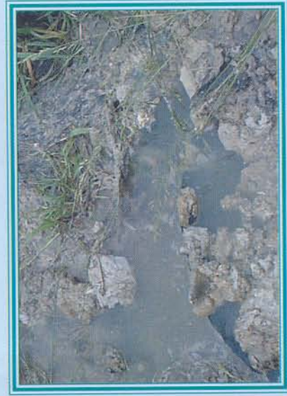
Improperly disposed grease waste overflowing from a sewer
