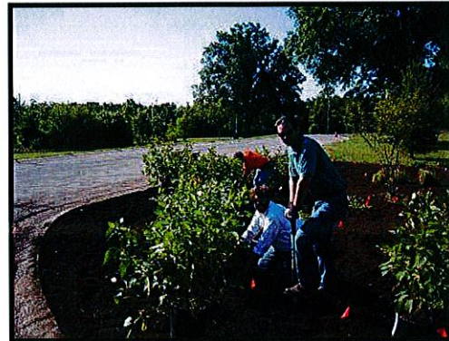
WSD Rain Garden Ground Breaking
